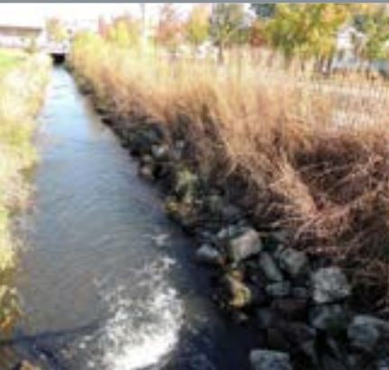
Stream Bank Stabilization
